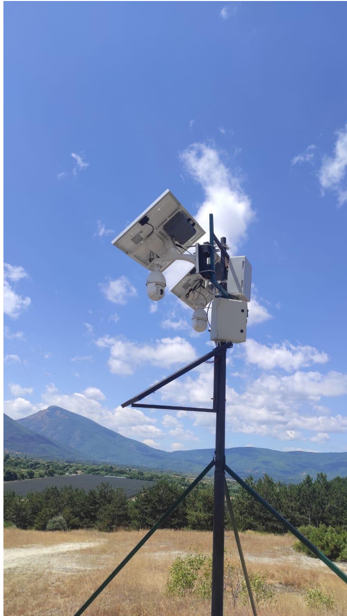
Figure 6: Camera system deployed at Rotino view point
