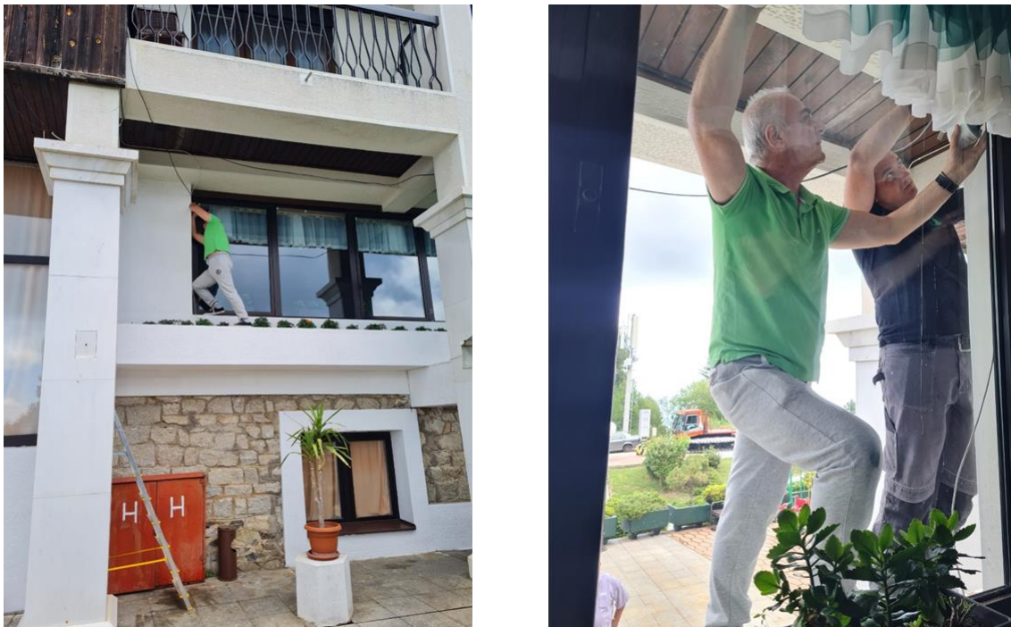
Figure 1 Installation of instruments at Molika (Pelister)
