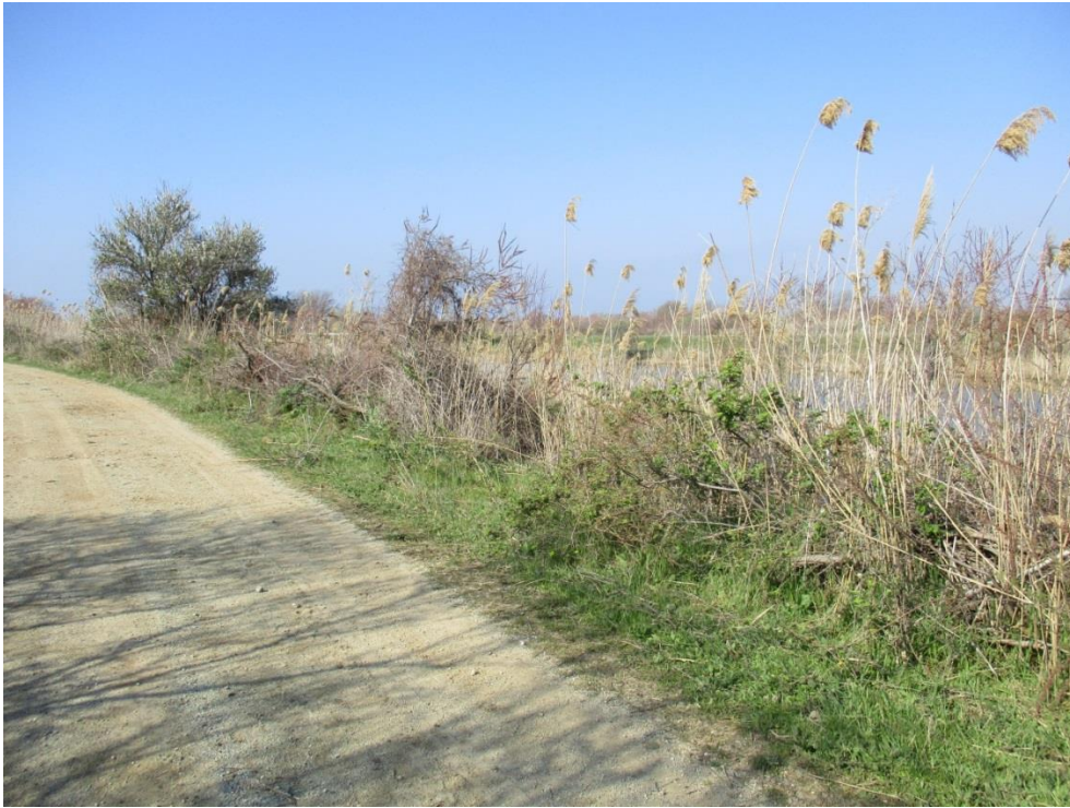
Photograph No 3: Embankment of Axios river canal
