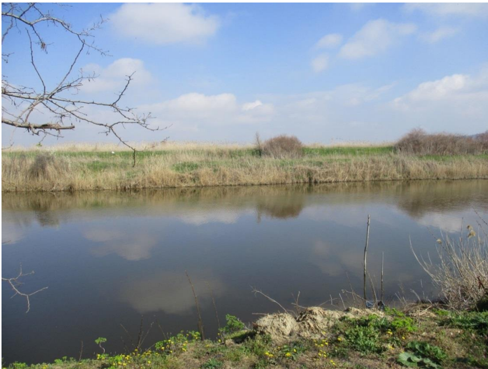
Photograph No 4: Embankment of Axios river canal
